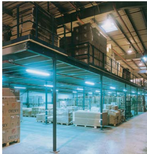
Warehouse mezzanine - pallet storage
