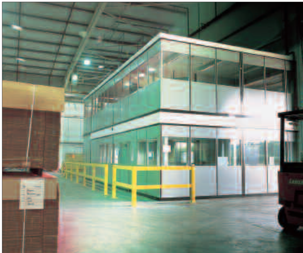
Steel partitioned two-storey office accommodation mezzanine
