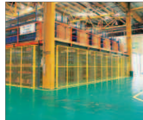
Secure storage factory mezzanine and steel screens
